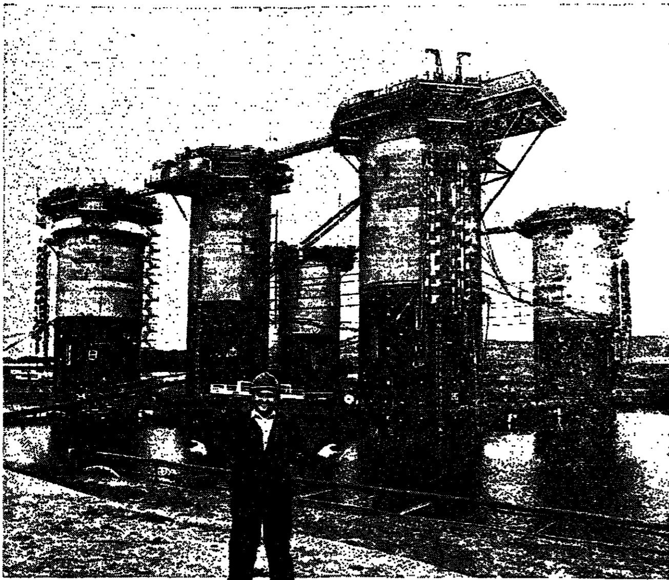
The massive Conoco TLP Hull just before tow-out from Hi-Fab's Nigg yard.
